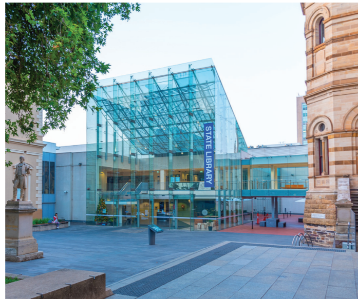
State Library Forecourt
